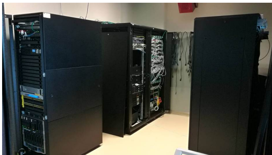
Figure 2. ICSTM Data Center (front: primary; back: secondary + distribution; right side: collocation).
