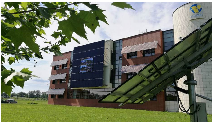
Figure 1. ICSTM BIPV (sun-shading, curtainwall and large array tracker) microgrid power source.
