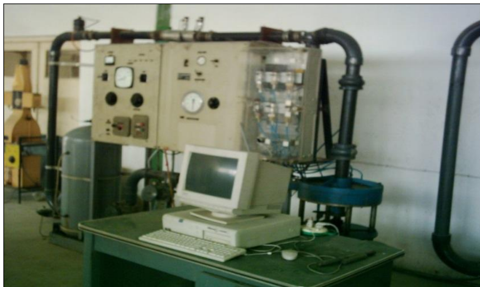
Figure 2. A centrifugal pump testing system.
